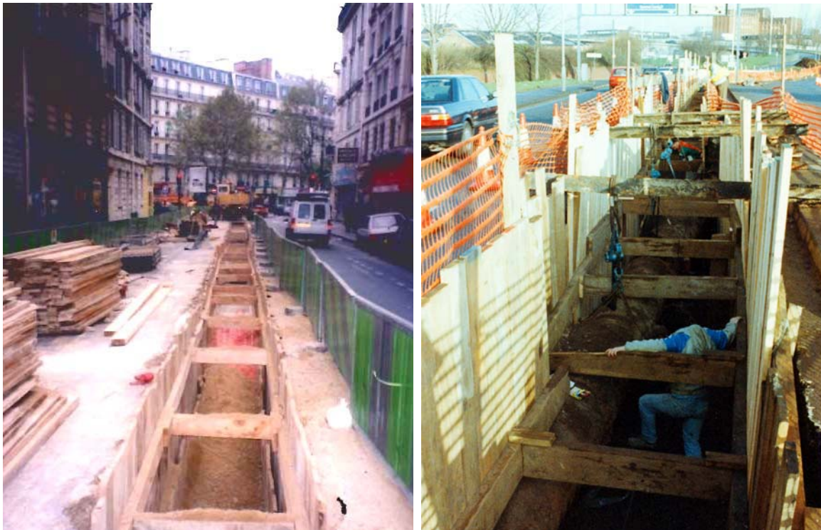
Figure 3.9: Trenches with shuttered (supported) walls
