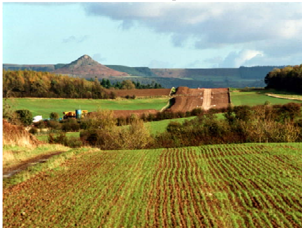
View of cable swath towards Roseberry Topping
