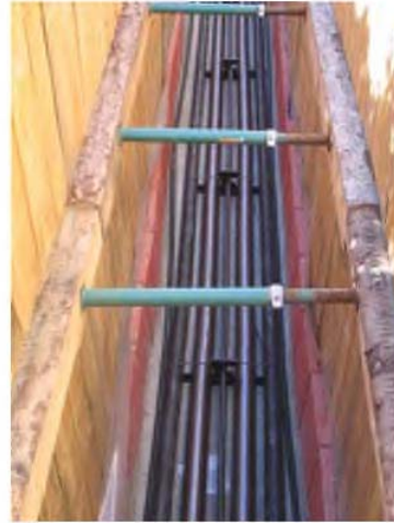
Fig. 3: Picture of the open trench under the pavement
