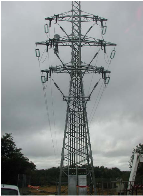
Figure 3.16 Tower-mounted terminations on a 90 kV line
