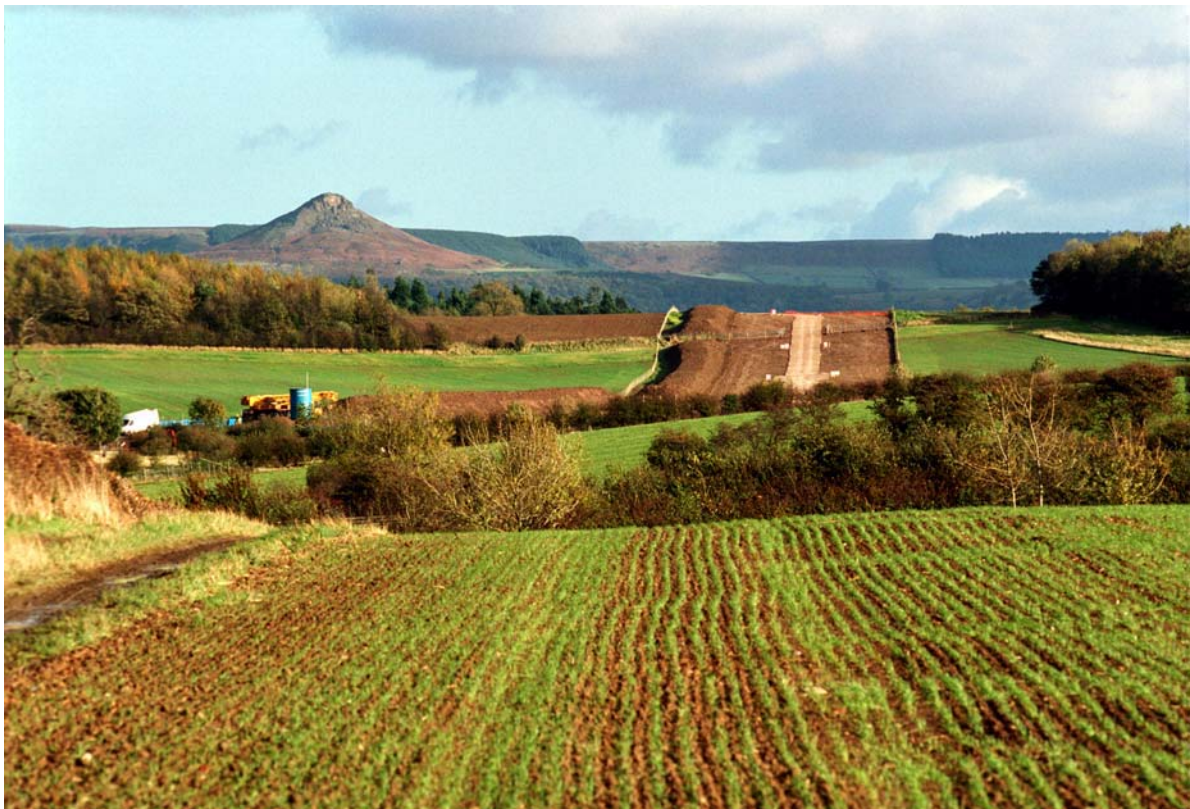
Figure 3.15 Construction swath for the Nunthorpe-Newby 400 kV cables in the UK. Further details on this installation are given in Appendix G.
