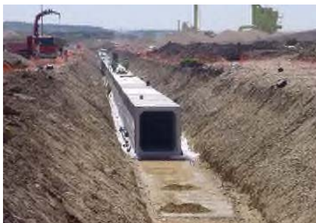
Tunnel under construction
